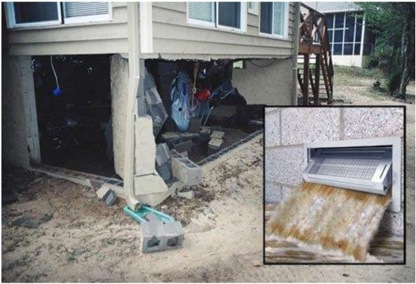
This floodproofing method involves adding openings beneath the lowest floor of your home to allow water to enter and exit in the event of a flood without causing structural damage. In the event of a flood, water can flow into and out of your home freely through the vents, with no need for human intervention, which will reduce the risk of structural damage to your walls or foundation.
