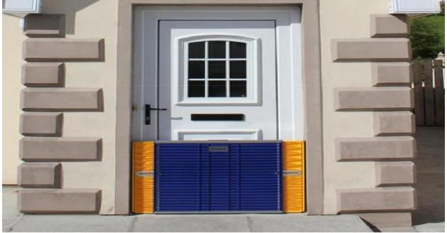
Sealing buildings to keep water out using passive or active mechanical devices such as concrete ring walls around a boiler, floodproof doors, or barriers.
