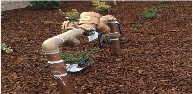
Backflow preventers stop sewer and stormwater from entering your home through sinks, toilets, and bathtubs when the systems surrounding your home are overwhelmed with flood water.
